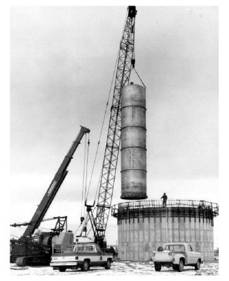
A tall steel cylindrical tank is being carefully lowered into a concrete silo by a crane during construction of the calcine storage facility.
