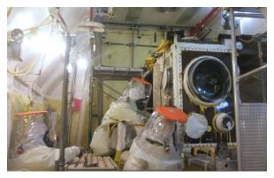
Sealing of one of the large 12' gloveboxes at the Hanford Plutonium Finishing Plant (PFP) in February, 2016.
