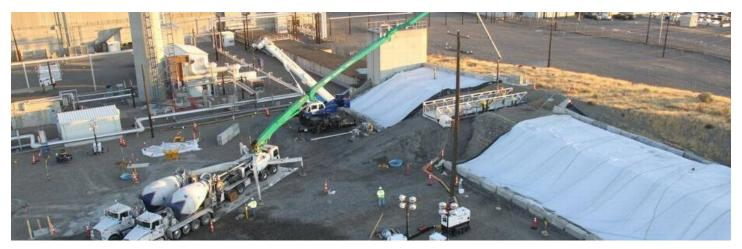
Grouting operation in November, 2017 to stabilize the smaller PUREX tunnel after a section collapsed.
