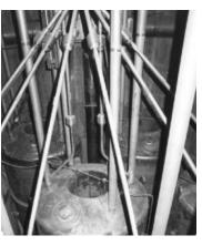
The interior view of a large concrete silo illustrates the complex system of pipes used to fill each of the four to seven cylindrical tanks within each silo.
