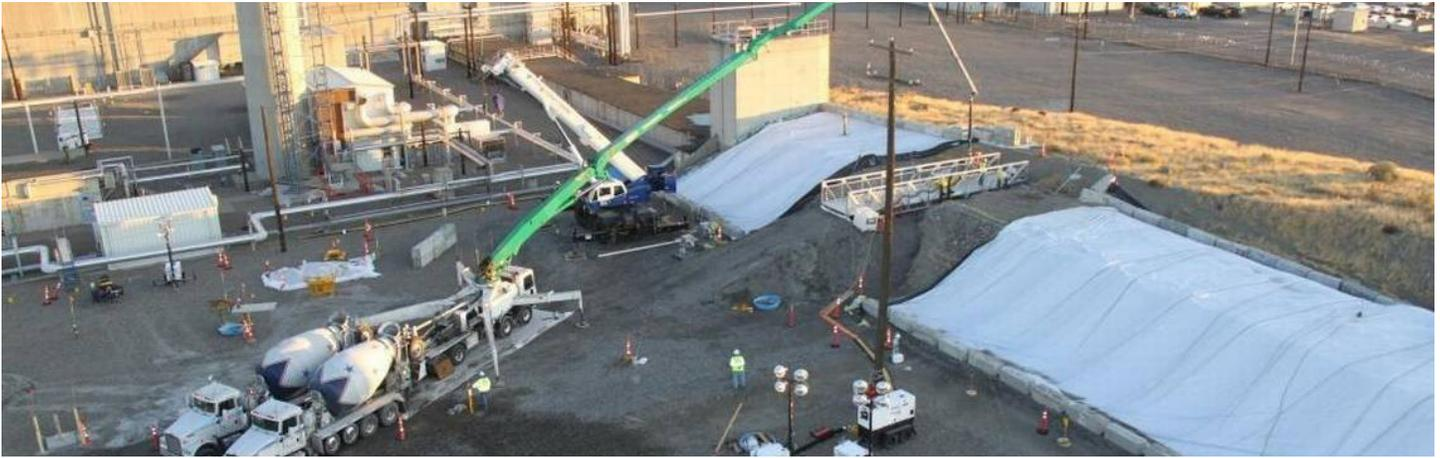
Grouting operation in November, 2017 to stabilize the smaller PUREX tunnel after a section collapsed.
