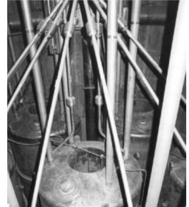
The interior view of a large concrete silo illustrates the complex system of pipes used to fill each of the four to seven cylindrical tanks within each silo.
