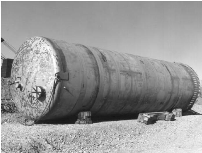
An unused steel cylindrical tank is shown prior to its insertion into a concrete silo. Fill pipes will be attached to the top of the tank while its base will be anchored to the floor of the concrete silo.
